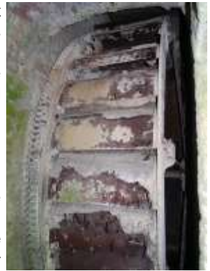
The gear teeth and buckets on the twenty foot water wheel.
